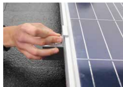
As you install each panel in the array check alignment and make minor adjustments as required. Once you have installed all panels in the array use End Clamp Kits to secure the last panel,
