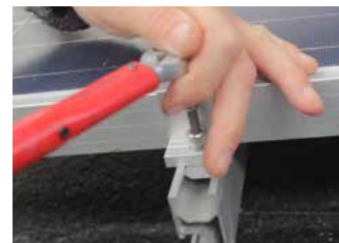
Hand tighten using a M6 Allen key and then use a torque wrench set at 15 Nm to tighten - check you have tightened ALL End Clamp Kits and Inter Clamp Kits in your panel array.
