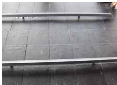
Now you are ready to mount the panel to the rail. Ensure rail ends are even at this stage. Extra Care must be taken with the first panel to ensure it is positioned correctly. This will assist in the even positioning of the final array
