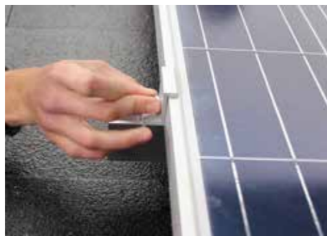
Lift panel onto the rail, sliding the End Clamp Kit on to hold it.
