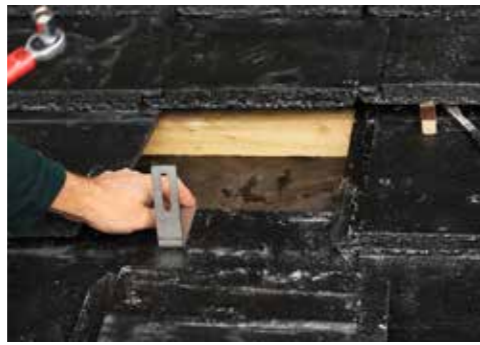
Sit the Solar Adjustable Tile Bracket on the tile in the desired location over the rafter.
