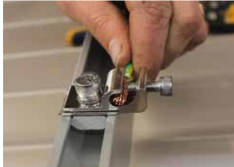
Clamp earth bonding wire between the screw in the Grounding Lug.
