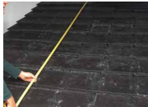
Begin by deciding the layout of the panel array in conjunction with the mechanical drawings supplied by the PV Install Designer. It is essential panels do not overhang spouting line or any roof lines.
