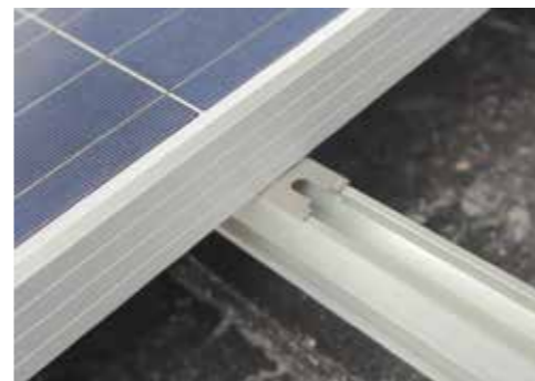
Before mounting the next panel Position your next Inter Clamp Kit and Grounding Clip ready for the next panel.
