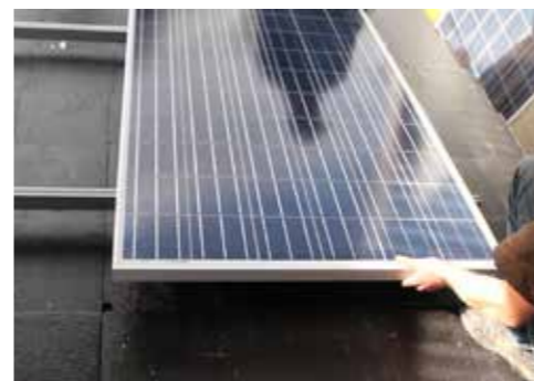
At this stage the panel alignment can be adjusted before the second End Clamp Kit is tightened. Ensure panels are following the correct line of the roof.
