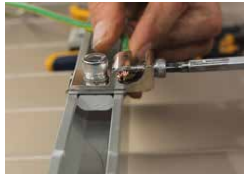
Tighten with M6 Allen key.
