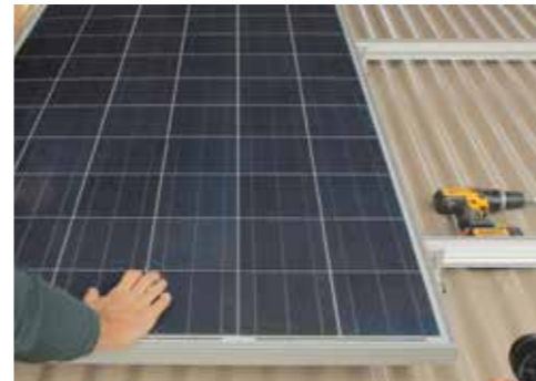
At this stage the panel alignment can be adjusted before the second End Clamp Kit is tightened. Ensure panels are following the correct line of the roof.
