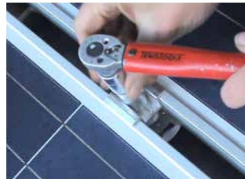
Check you have tightened all nuts with a torque wrench set at 17.5 Nm
