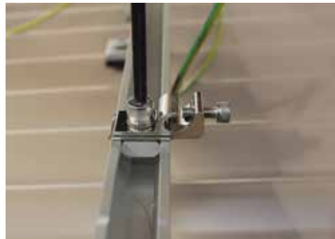
Insert Grounding Lug into rail by sliding it in. Tighten with M6 Allen key.
