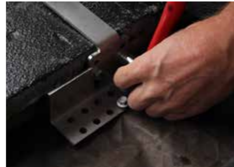
Once the bracket is in position, set a torque wrench to 15Nm and tighten the M8 Stainless Steel nut & bolt assembly
