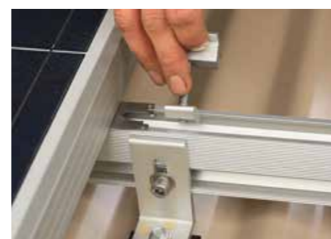
Before mounting the next panel position your next Inter Clamp Kit and Grounding Clip ready for the next panel.
