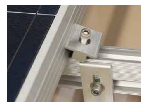
Carefully position next panel - take care to ensure the Grounding Clip is flat and level. Once flat push the two panels together and hand tighten using a M6 allen key
