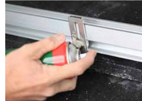
Spray lanolin liberally on all stainless and aluminum interface connections for long term corrosion resistance
