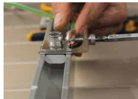
Set up the earth connection on the rails following the steps demonstrated in Section 1: Demonstration of Earthing using Grounding Lug in this Installation Guide, in conjunction with the mechanical drawings supplied by your PV Install Designer
