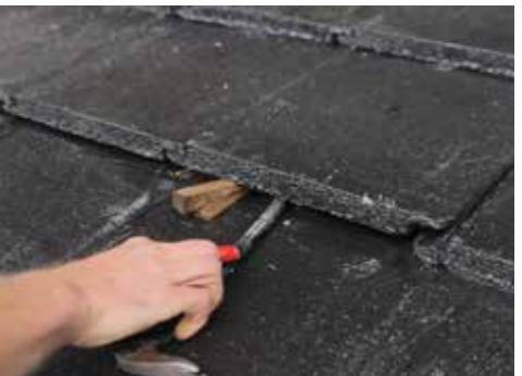
The Solar Adjustable Tile Bracket sits underneath the tiles and fixes to the roof rafters. Once the position of panels is decided you must establish where the roof rafters lie underneath the tiles, generally they are 900mm apart.
