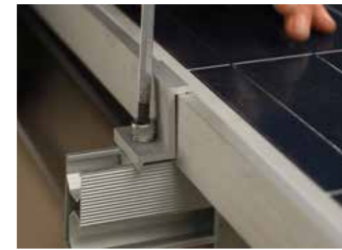
Use a M6 allen key to hand tighten
