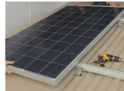
Lift panel onto the rail, sliding the End Clamp on to hold it.
