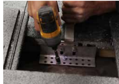
Use two M6 wood tech screws that come with the Solar Adjustable Tile Bracket Kit to fasten the bracket on to the rafter.
