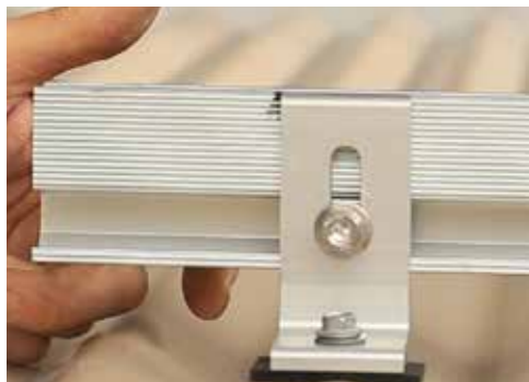
Mark the top of the rails where the edge of the panel will sit, this is typically 50mm in from the ends.
