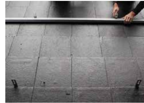
Rest the rail you cut to length earlier on the roof brackets while you position the Tilt-In Set bolts - these bolts are included in the Solar Adjustable Tile Bracket Kit.
