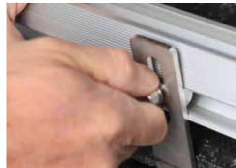
Attach the Tilt-In Set bolts loosely to the bracket riser, then maneuverer the Slide Nut into the slot of the rail - if bolts are difficult you can leverage gently with an allen key.
