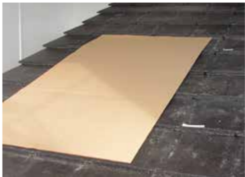
When you have decided on the position of your array, mark the position of where the brackets will go using tape or a marker pen.
