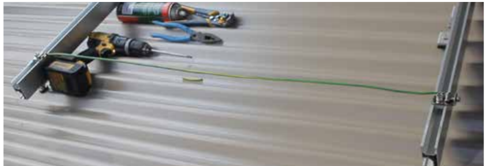
Run the earth wire down to the next level of rail and install another Grounding Lug following the same procedure
