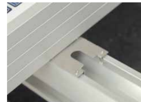
These are installed between the panel and the rail using the Inter Clamp Kit . It is ESSENTIAL care is taken in this step to ensure a quality earth.
