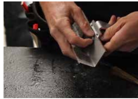
There is both vertical and horizontal adjustment in the bracket to suit the profile of the roof tile.
