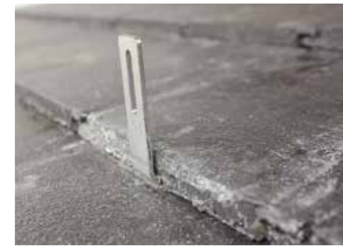
The first bracket is now ready for rail to be mounted to it, Repeat this process to mount the next brackets in your PV System Design
