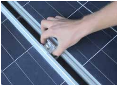
When the S-5 PV Kit Bracket is used as an Inter Clamp Kit the bottom Riser Nut is not required
