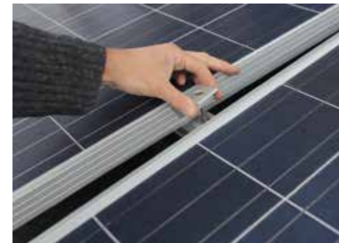
Carefully position next panel - take care to ensure the Grounding Clip is flat and level. Once flat push the two panels together and hand tighten using a M6 allen key
