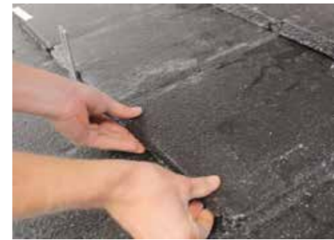
Replace the tile you have ground the slot out of and any other tiles you have removed next to it.
