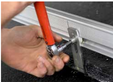
Tighten by hand using a M6 allen key and once all rails are installed and you are happy with your rail height use a torque wrench set at 15 Nm and tighten.
