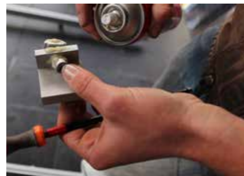
Set up the earth connection on the rails following the steps demonstrated in Section 1: Demonstration of Earthing using Grounding Lug in this Installation Guide, in conjunction with the mechanical drawings supplied by your PV Install Designer
