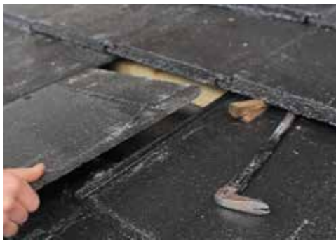
Once a tile is removed you can confirm the rafter position
