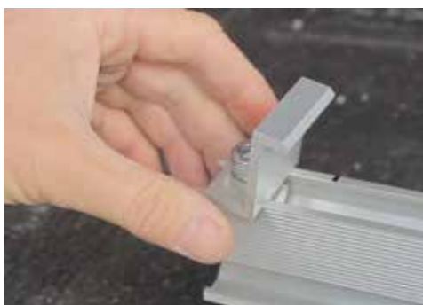
Loosely position End Clamp Kit where you have marked on the rail.
