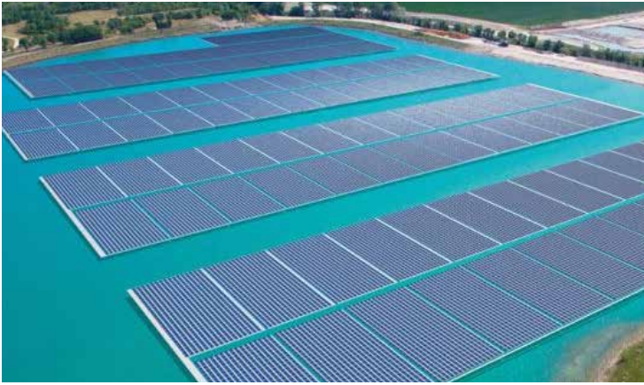
Image: French Floating Trina Solar PV modules
